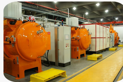
Heat treatment workshops
